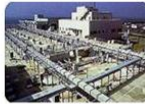
Sewage Treatment Center
